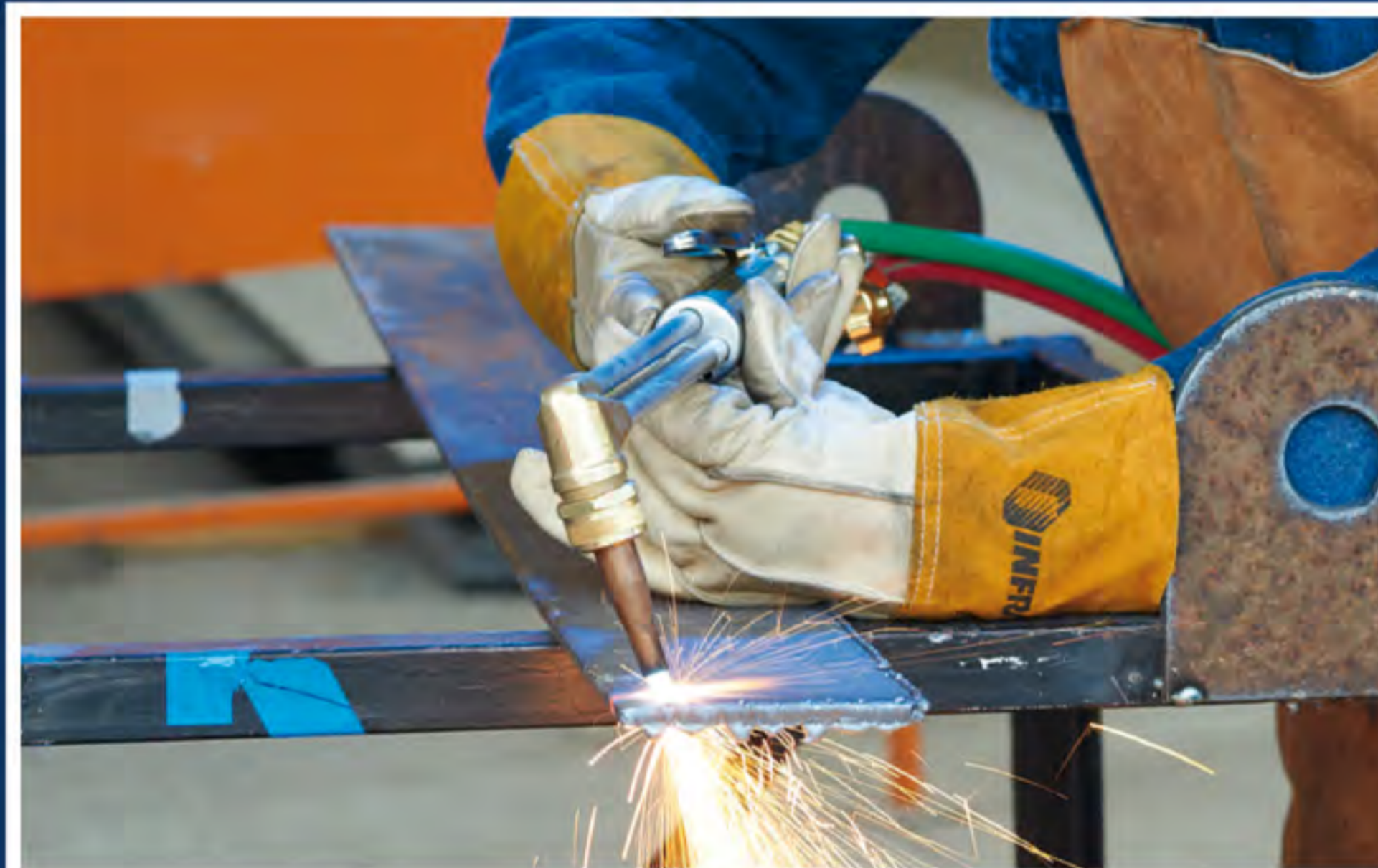
Oxyfuel Welding and Cutting
